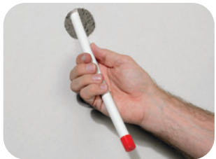
Figure 28: Always protect pipe ends
