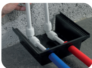
Figure 46: Cut conduit box for wall termination
