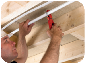
Measure and cut in-situ
