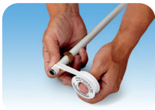
Apply PTFE tape if required
