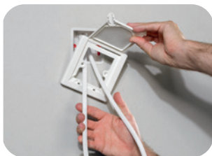
Figure 58: Installation procedure of HX113 cover plate
