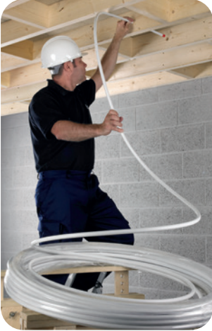
Figure 29: Packaging retains pipe until last metre
