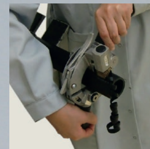
Scrape and degrease the pipes
