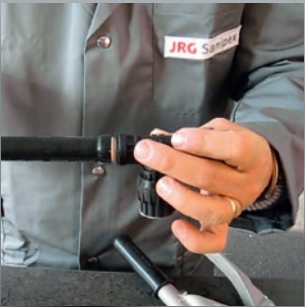
Insert the expanded pipe into the fitting
