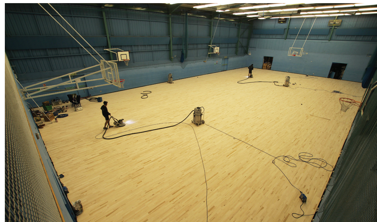
The new MVP floor is given a light sanding before the application of a Bona Supersport sealer
