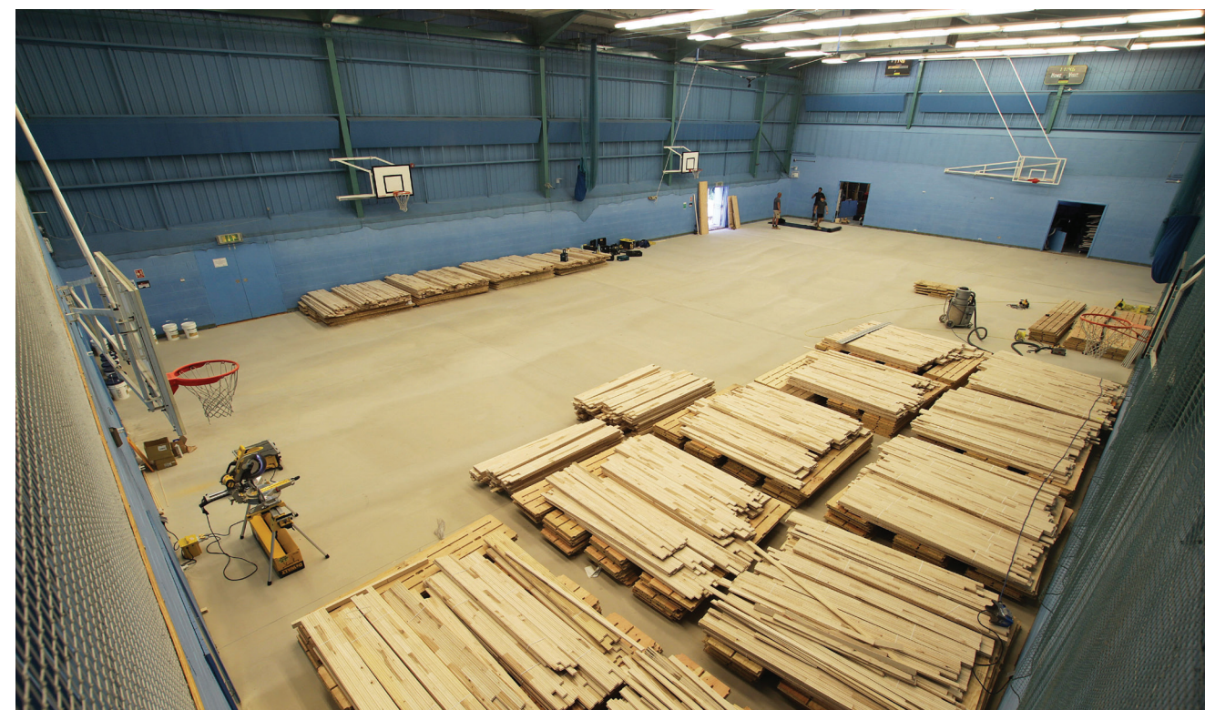
The substructure of the University's old court was refurbished before the new flooring could be laid
